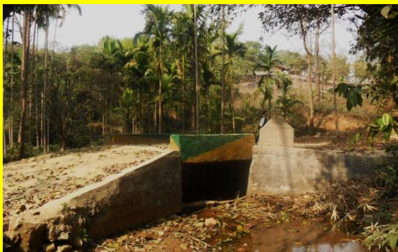
Causeway/Culvert at Dawa m/watershed, IWMP-I
