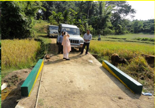
Causeway/culvert at Dawa m/watershed, IWMP-I
