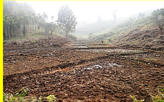
Bench Terracing at Songgitchak m/watershed
