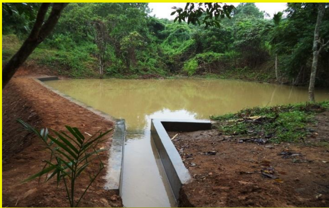
Water Harvesting Structure at Jembra Nomil Asi m/watershed, IWMP-IV
