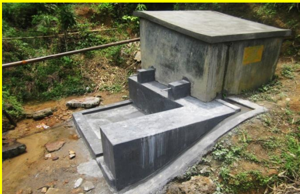
Improvement of Spring Chamber at JembraNomilAsi,
