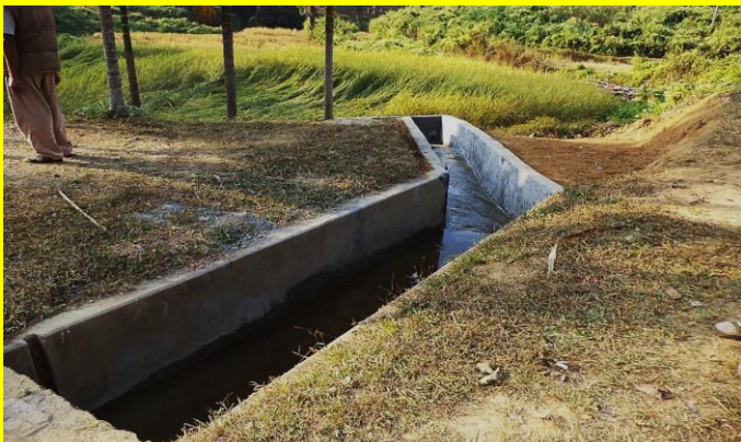
CC Irrigation Channel and Earthen Irrigation Channel at Chenggal m/watershed, IWMP-II
